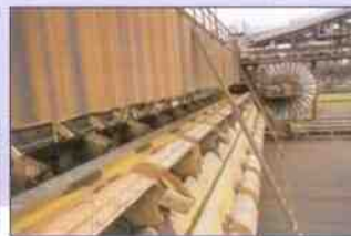
Bridge Type Drum Reclaimer
